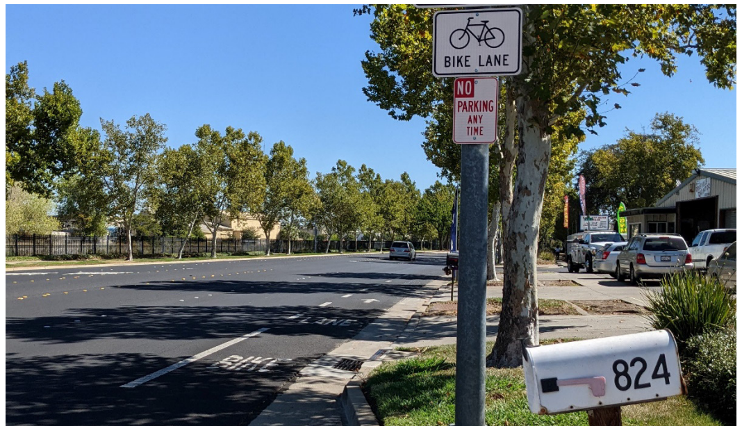
Existing Class II bike lanes on Atlantic Street.
